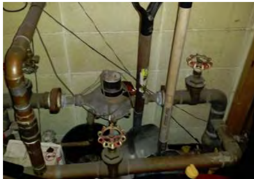
Figure 1: No Backflow Device @ Water service
