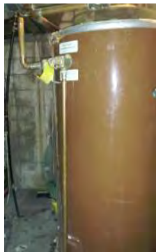
Figure 2: Domestic Hot Water Tank
