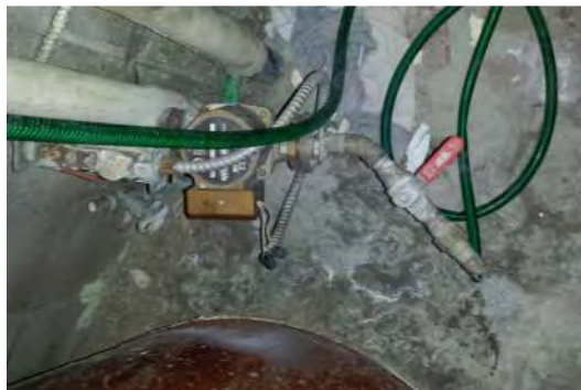
Figure 3: Domestic Hot Water Tank Disconnected Recirculation System
