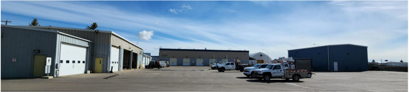
Figure 3: Interior View of the Fort Saskatchewan Public Works Yard
