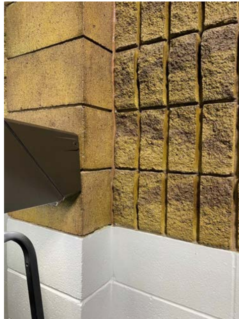
Photo 2: Caulked joint on east wall
