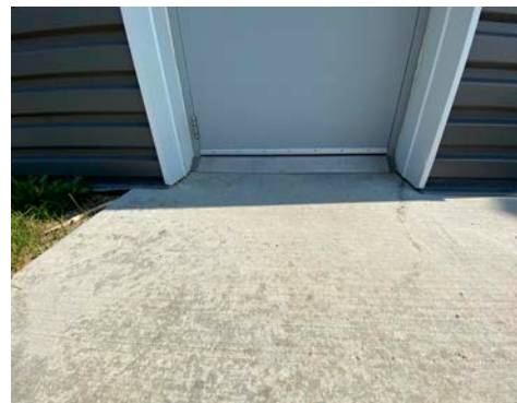
Photo 15: Exit Door with significant slope transition
