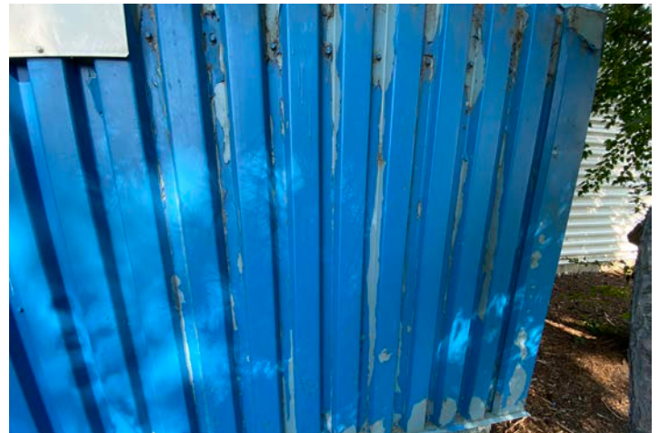
Photo 8: Delaminated Cladding
