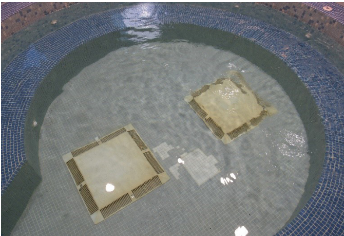
Dual main drains in the whirlpool.
