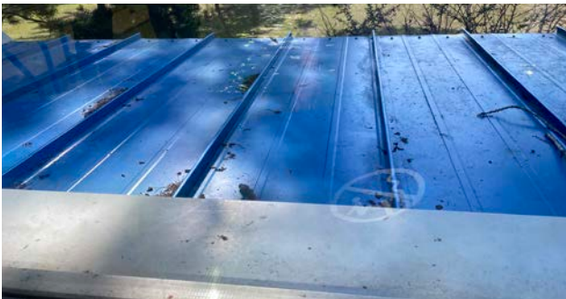
Photo 6: Standing Seam Roof
