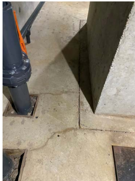
Photo 8: Cracking in the basement slab-on-grade
