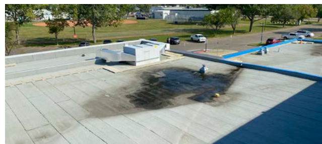
Photo 9-10: Ponding on Roof
