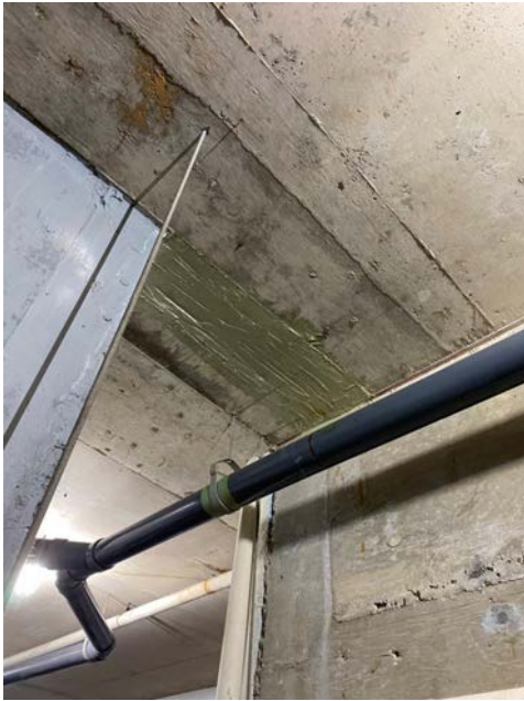
Photo 5: Repaired crack in storage room
