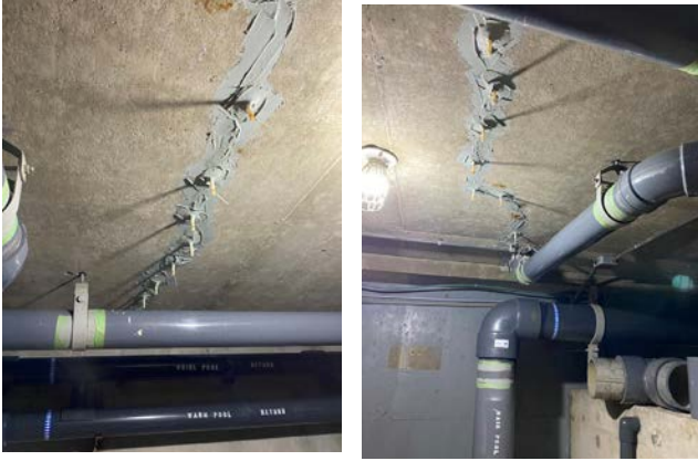
Photo 3 & 4: Repaired cracks on the underside of the pool deck structural slab
