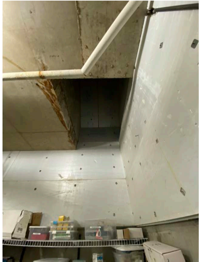
Photo 56: Water Staining
