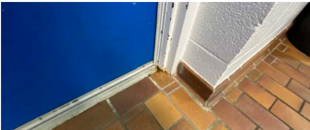
Photo 17: Corrosion on Doors
