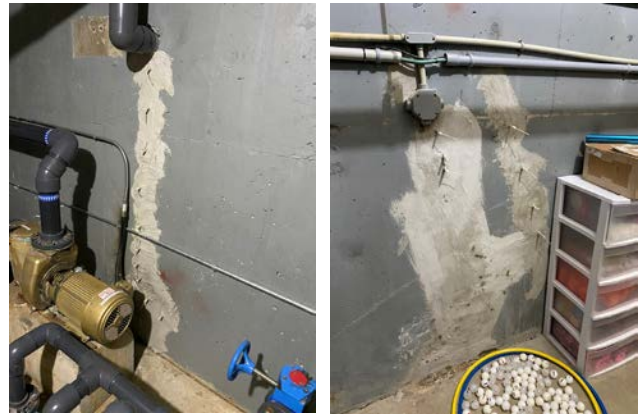
Photo 6 and 7: Repaired cracks in the pool tank walls
