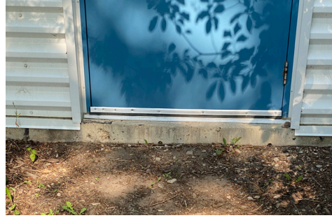
Photo 13: Exit Door with significant drop
