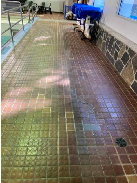
Photo 40: Delaminated Floor
