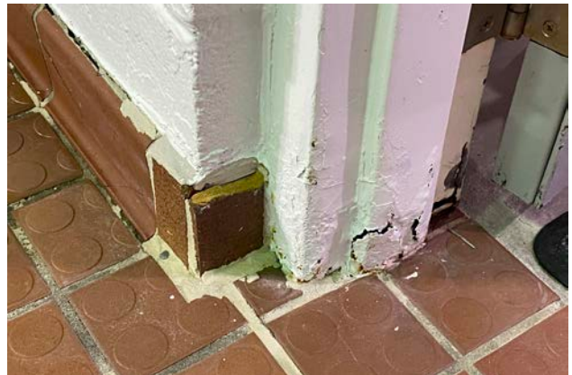
Photo 43: Corrosion on Door Frame
