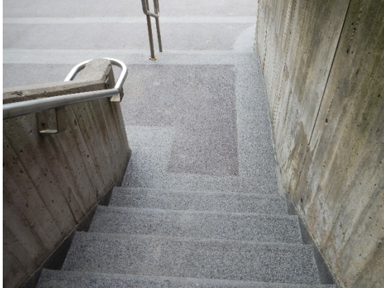
Example of Stone Grip System on Stairs
